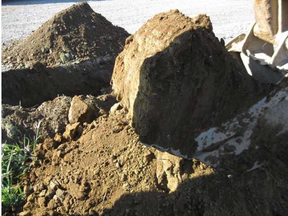
Photo 5 - TP-1 Excavation Material
