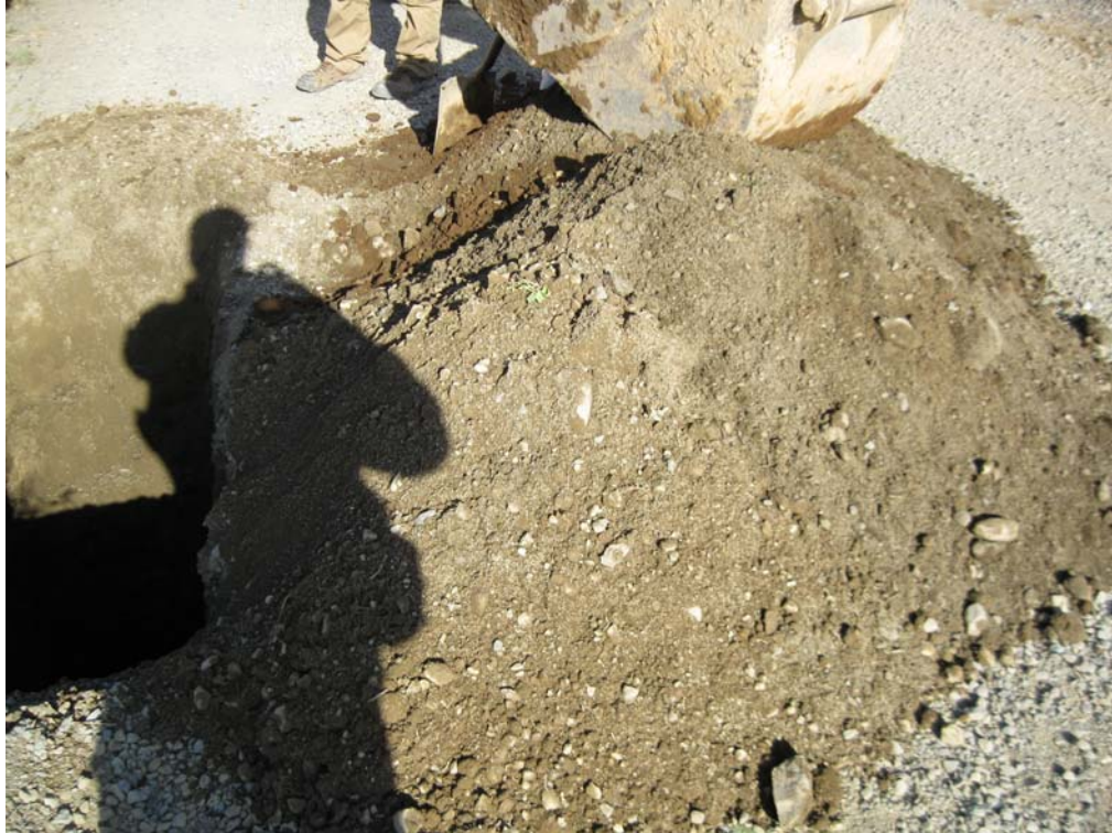
Photo 25 - TP-7 Excavation Material
