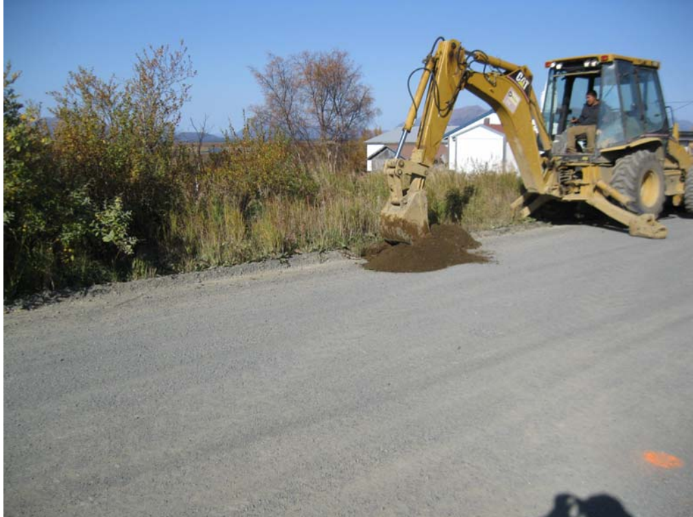
Photo 10 - TP-3 Test Pit Location
