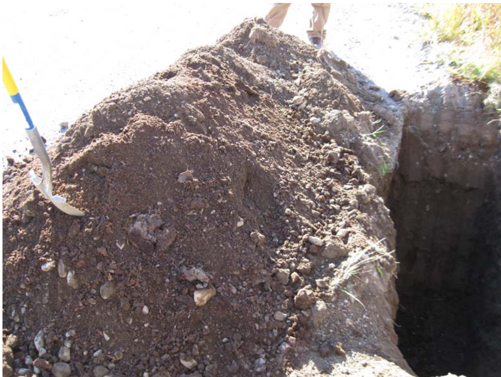
Photo 12 - TP-3 Excavation Material
