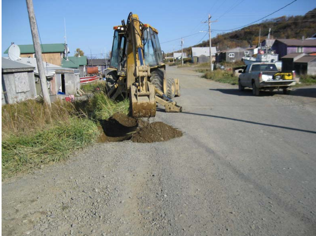
Photo 6 - TP-2 Test Pit Location
