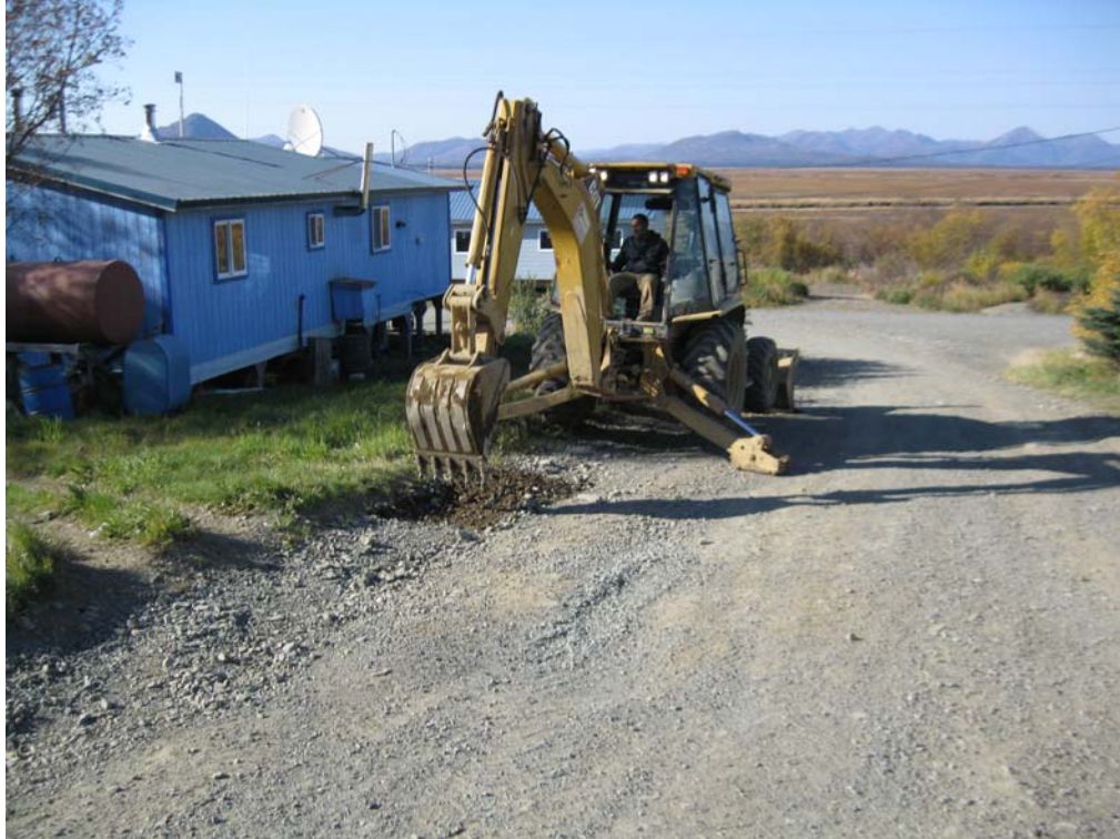
Photo 13 - TP-4 Test Pit Location
