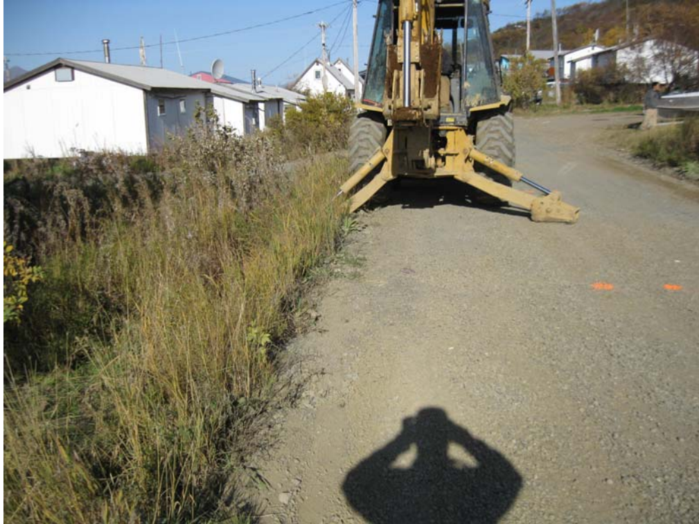
Photo 23 - TP-7 Test Pit Location
