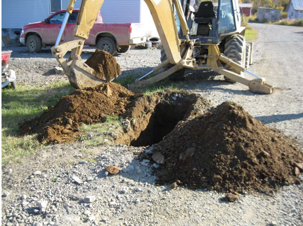
Photo 2 - TP-1 Test Pit Location
