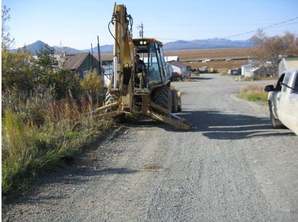
Photo 20 - TP-6 Test Pit Location
