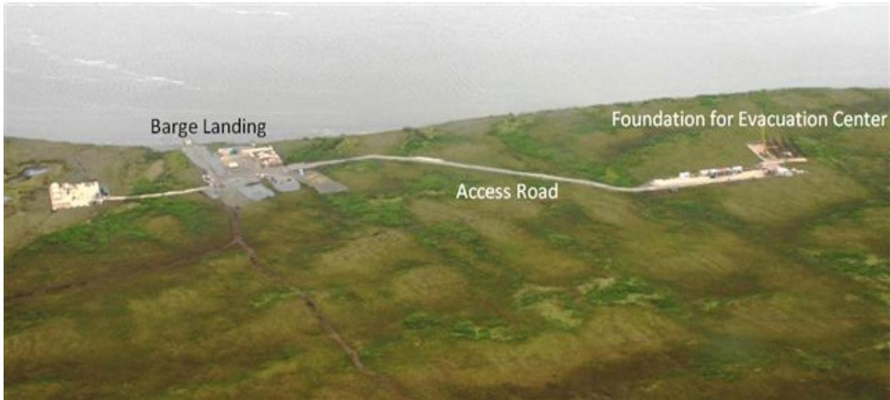
Figure 1. The beginning of a new village--Mertarvik Barge landing, Access road and evacuation center foundation (right). Photo: Harvey Smith, DOT/PF
