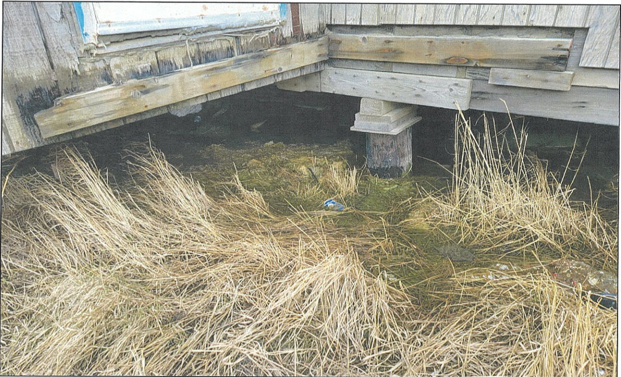
IRA Building – Wood sleepers above wood pile
